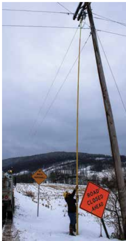
REPAIRS UNDER WAY: Jeremiah Lund, a journeyman lineman with Claverack’s Wysox District, uses a hotstick to close in a circuit and restore power to members in Bradford County Jan. 4. Accumulations of wet, heavy snow the night before made accessing co-op lines challenging in some of the remote and higher-altitude locations of the co-op’s service territory.
