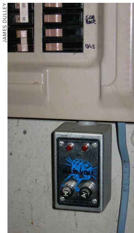
SURGE PROTECTION: This whole-house surge suppressor is mounted beneath the circuit breaker panel in Jim Dulley's house.
