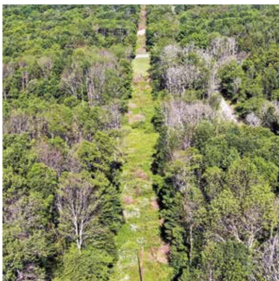
BIRD'S EYE VIEW: Aerial photographs taken from a drone last summer show numerous dead ash trees lining co-op right-of-way corridors in Bradford County. The majority of 2021's unprecedented number of tree-related outages were caused by standing dead ash trees like these. Although located outside the co-op's standard 40-foot rights of way, the brittle trees are tall enough to topple onto co-op lines during high winds.
