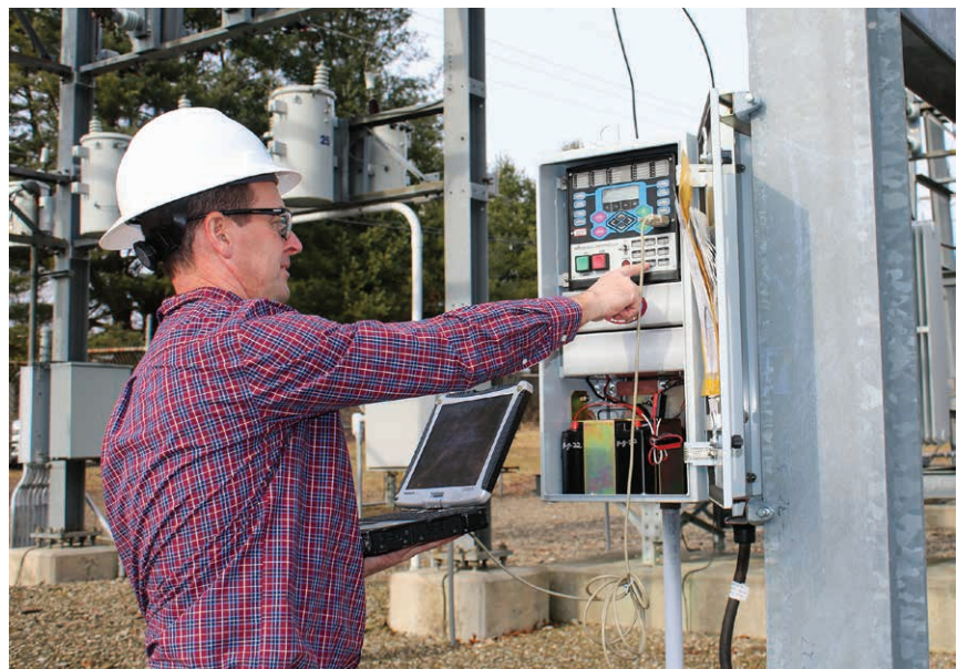
REMOTE CONTROL: Claverack REC's technical services supervisor, Larry Beebe, uses a tablet to operate a recloser controller at the Lime Hill Substation. The fiber-optic network Claverack is constructing will give the cooperative improved capabilities for remotely controlling devices in the field from the office.
