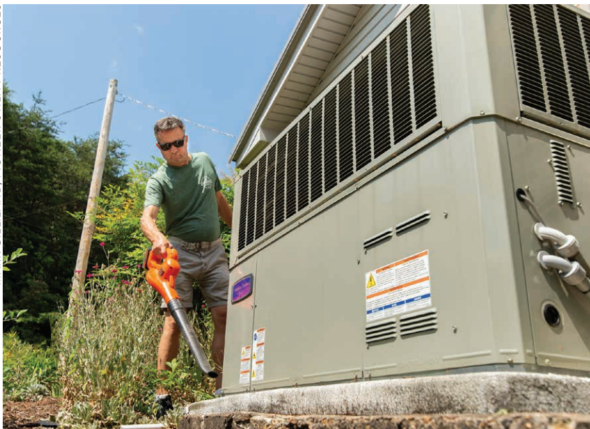
A LONGER LIFE: The lifespan of a heating and cooling system ranges from 15 to 20 years. Proper maintenance and lower use can increase the life of the equipment.
