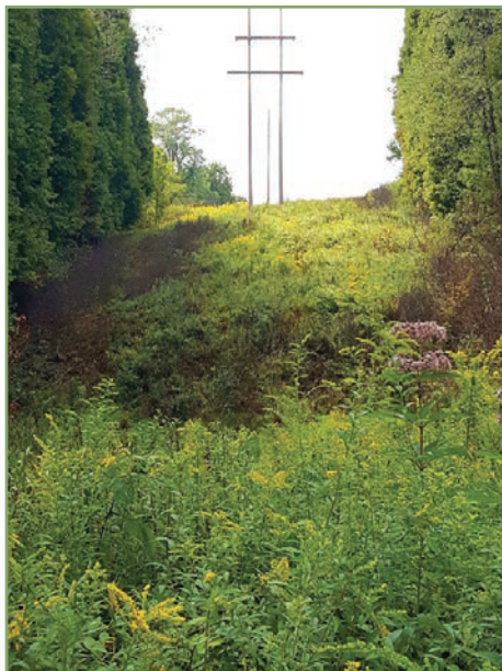
This electricity transmission R-O-W is well-established with beneficial native grasses, such as deertongue ( Panicum clandestinum ), and forbs including various goldenrods ( Solidago spp) and Joe Pye weed ( Eupatorium fistulosum ).
