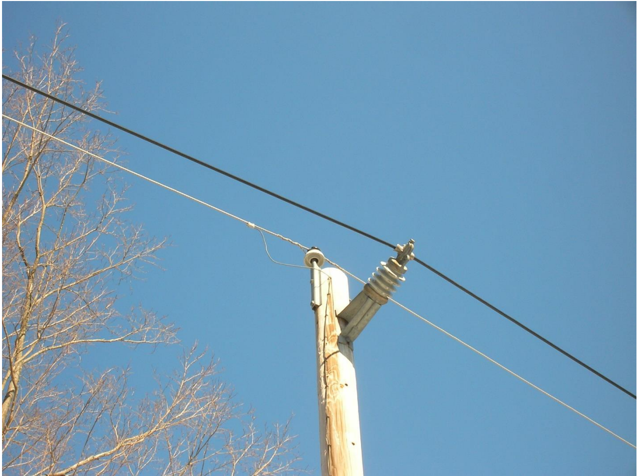
SINGLE SUPPORT, HORIZONTAL POST INSULATOR, TREE CABLE
